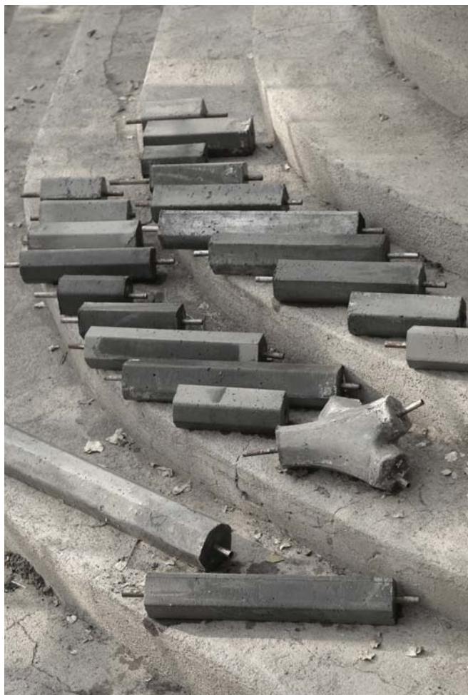
10 Prefabricated elements and nodes prepared for assembly.
