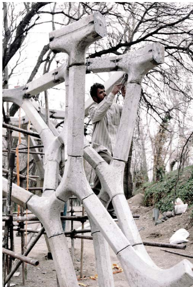
11 Constraining the compressive members with the tensile members in assembly.
