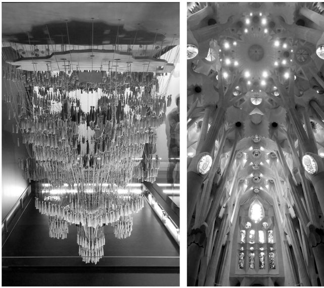
Fig. 1. Left: Physical form finding by Antoni Gaudí; and Right: The Basílica de la Sagrada Família's funicular structures designed by Gaudí (photo credit: authors, 2019).
