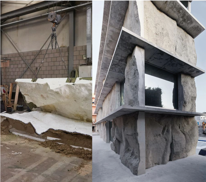
Figure 3: sand-casted concrete facade clads Anne Holtrop's green corner building in Bahrain (Holtrop, 2020).
