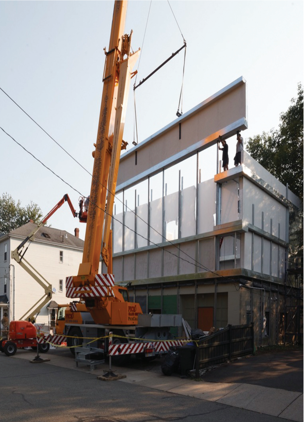
Ensemble studio, Cyclopean house construction, Cambridge, United States.
