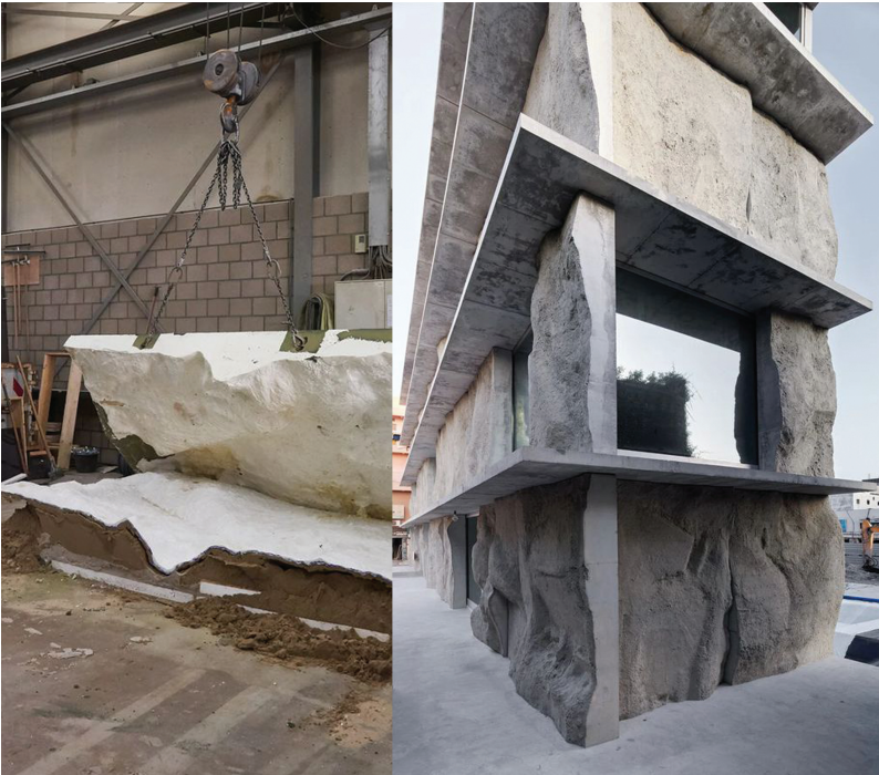
Figure 3: sand-casted concrete facade clads Anne Holtrop's green corner building in Bahrain (Holtrop, 2020).
