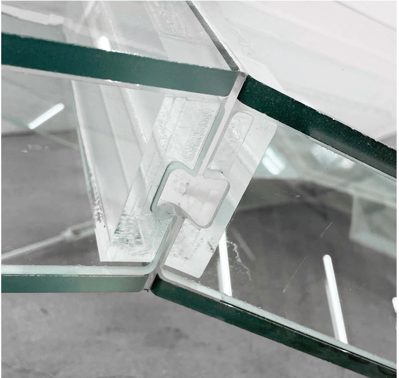
4 Close-up of the butterfly connection mechanism
