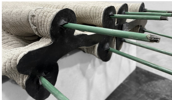
(b) Threading cables
