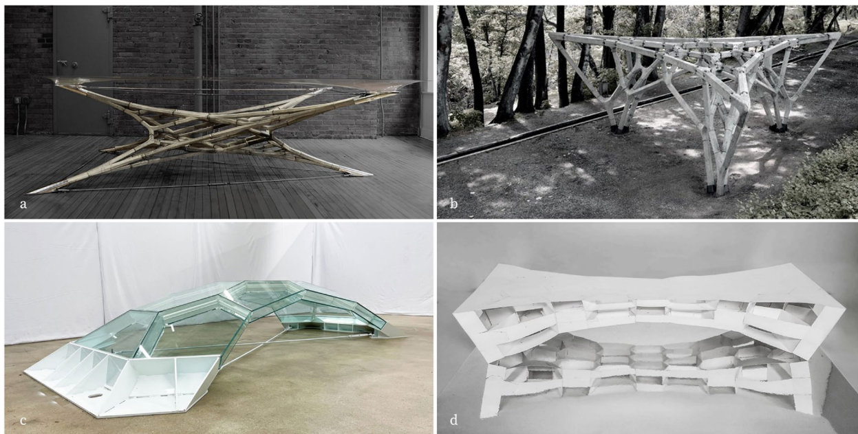
Fig. 2 Built projects designed with polyhedron-based 3D graphic statics: (a) a concrete spatial table (Akbarzadeh et al., 2021); (b) a concrete pavilion (Bolhassani et al., 2018); (c) a glass bridge (Lu, Seyedahmadian, et al., 2022); and (d) a paper bridge (Lu, Alsalem, & Akbarzadeh, 2022)
