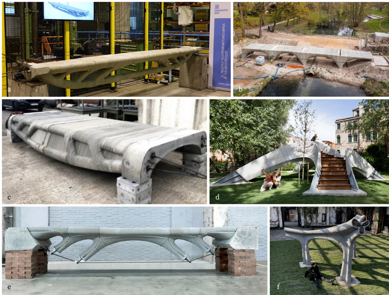
Fig. 1 Discrete 3D printed architectural systems: (a) Post-tensioned concrete beam (Vantighem et al., 2020); (b) Multi-span post-tensioned concrete bridge (Ahmed, Wolfs, Bos, & Salet, 2022); (c) Post-tensioned concrete bridge (Ooms et al., 2022); (d) Unreinforced concrete masonry footbridge (Bhooshan, 2022); (e) Post-tensioned concrete bridge (Li et al., 2024); and (f) Post-tensioned concrete pavilion (Wu et al., 2022)
