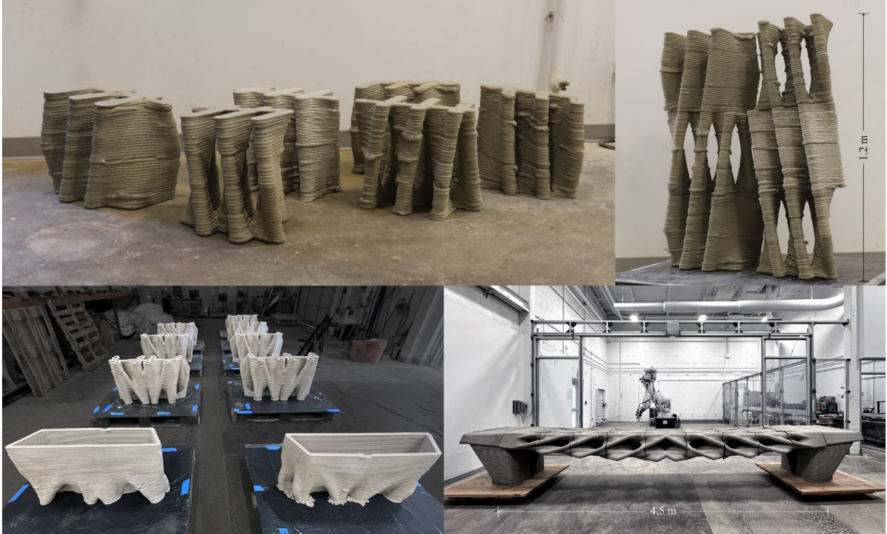
Figure 21: Top: a 3D-printed concrete wall with 6 components whose bridging points were reinforced by custom curves [6]. Bottom: a post-tensioned 3D-printed concrete canopy with embedded anticlastic geometry whose 9 components were optimized to reduce overfills while the conduits for post-tensioning were preserved [5], [39].
